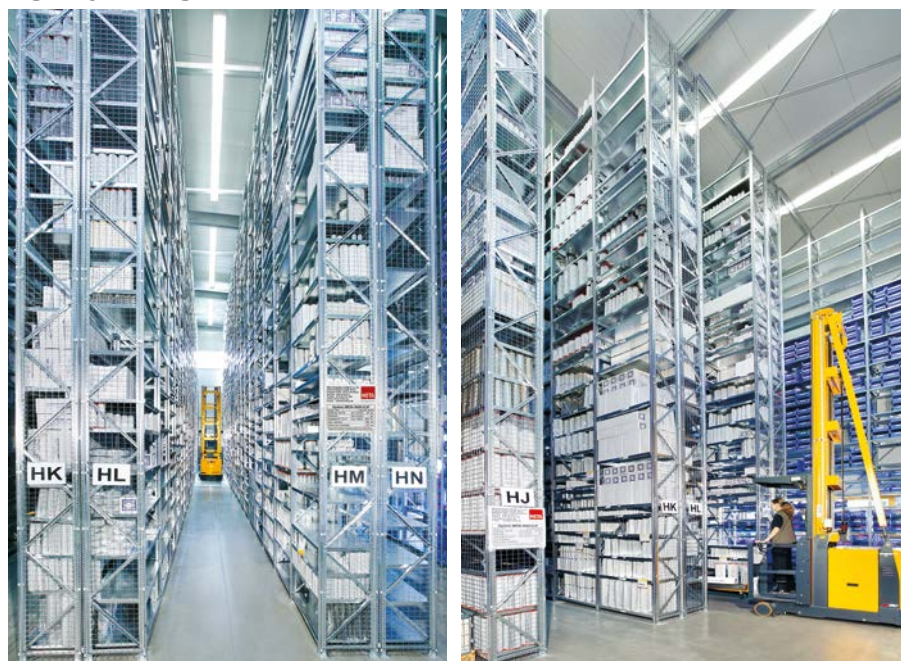
Fachboden-Hochregal High-bay shelving
